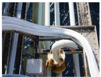
CharCoat CC forms a protective intumescent char when exposed to flame or to a temperature above 175°C. This char should be removed completely and clean cables should be recoated if intumescence should occur. There is no need to replace cable that has been subjected to fire as CharCoat CC sacrifices itself to save the cable (as long as the cable is functioning).
